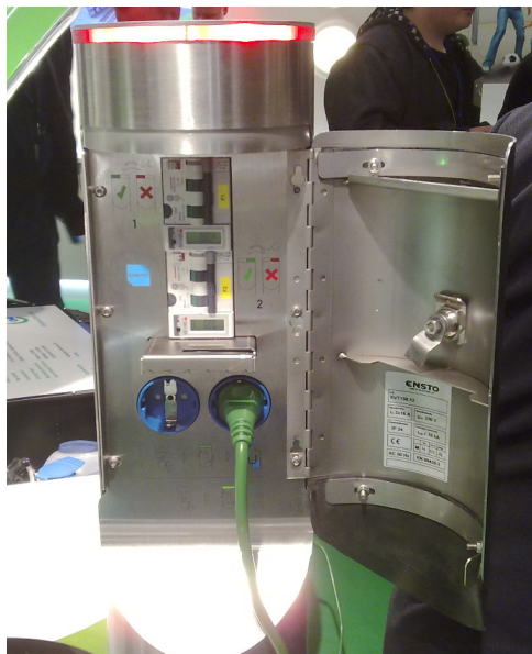
Figure 9: Charging station with kWh-metering by Ensto
