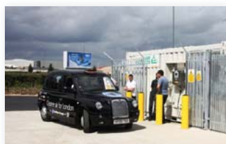
Heathrow Airport – Air Products – Opened August 2012
