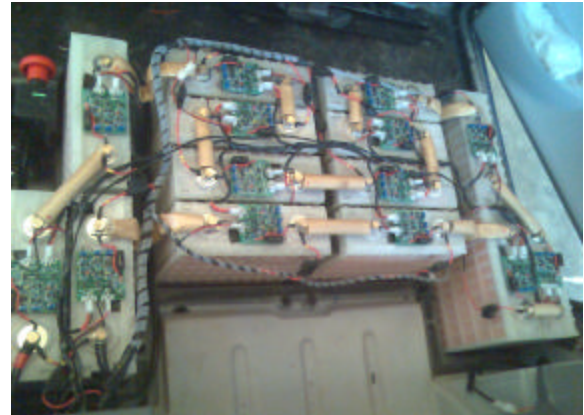
Fig 5. Lithium Battery pack with local monitoring
