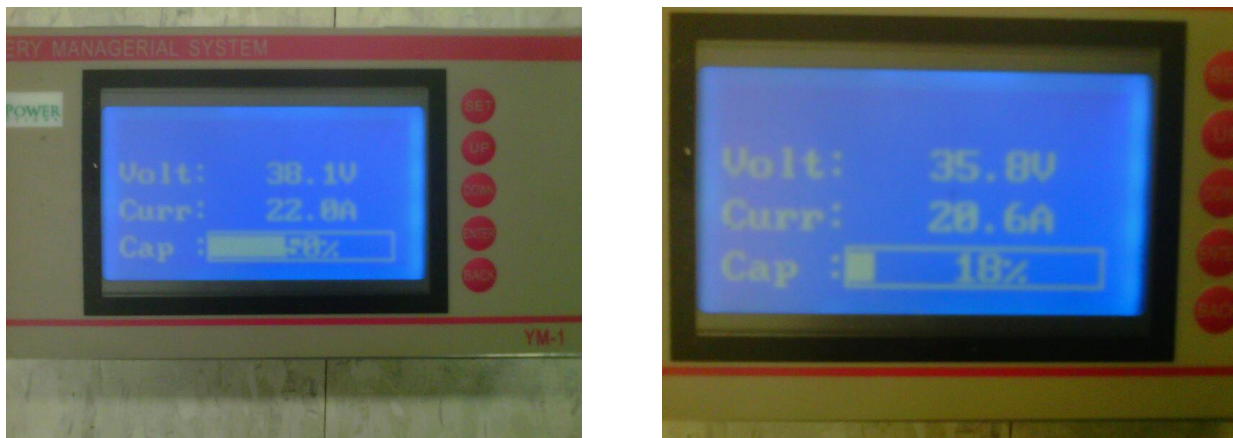
Figure 5.6. BMS displays at 50% charge (Left) and 18% charge (Right).
